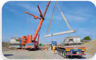
(Bridge Beams being placed)
